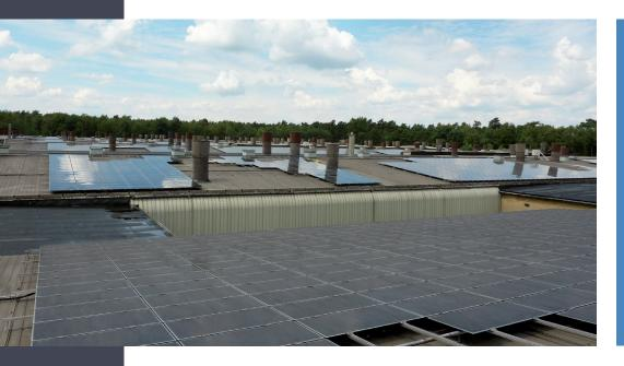
QLEEN has proved of value under the most difficult operations. This very large plant with an inclination of only 12 degrees exposed to atmospheric conditions as well as to the chimneys of a mast operation. Tenacious dirt forms quickly and cleaning is often necessary. Despite of much care the yield is OK.
